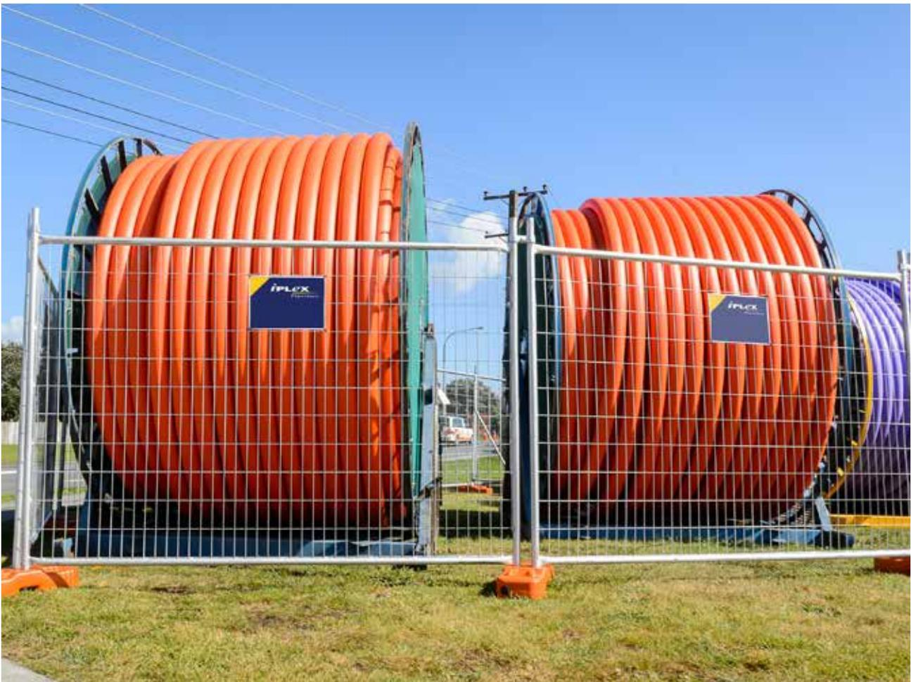
Image 11. Drum Coils safely stored on site in a fenced off restricted area.
