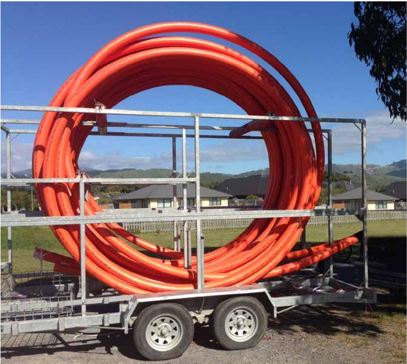
*Image 9. Large free standing electrical duct coils on a frame style dispensing trailer.*
