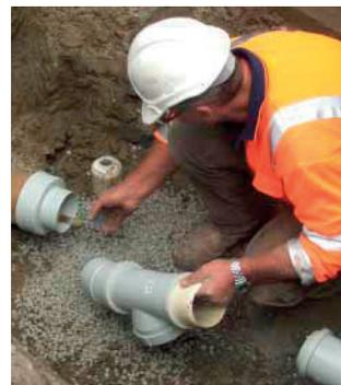
Installing DN100 Iplex NOVADRAIN® pipe with coupling and inspection pipe fitting, Christchurch City.
