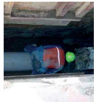
Deep installation of Iplex NOVADRAIN® DN300 SN4 at 4.8m cover under main road, Gisborne City.
