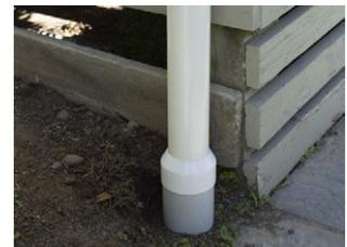
*Note: Iplex® recommend the installation of a PVC DWV access junction with sealed removable access cap, - positioned near to ground level, in "charged" inverted syphon pipes connected to rainwater tanks, to aid periodic flushing of the charged pipe.*
