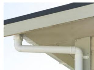
Support the offset by installing a pipe bracket directly below the lower offset bend.
