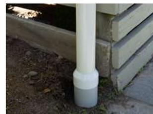
*Note: Iplex® recommend the installation of a PVC DWV access junction with sealed removable access cap, - positioned near to ground level, in "charged" inverted syphon pipes connected to rainwater tanks, to aid periodic flushing of the charged pipe.*
