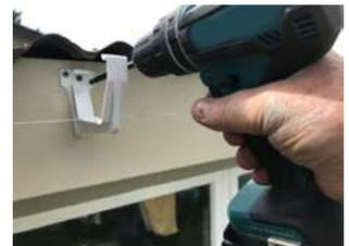
**NB. Corrosion resistant screws must be used, such as stainless steel or epoxy coated, suitable for treated timber.**
