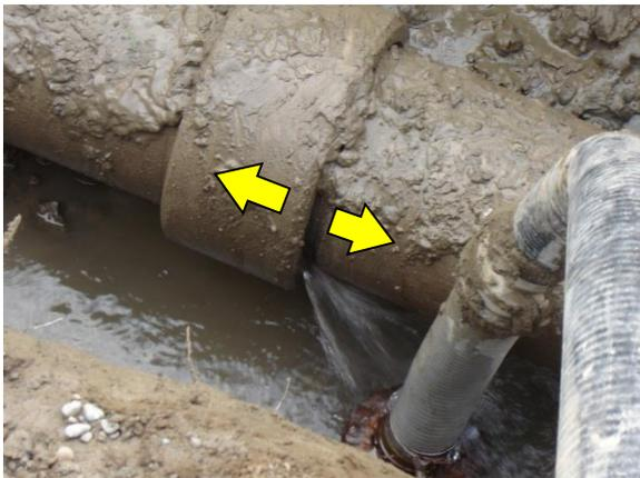
*Figure III - Tension effects in AC pipe joint, Sewell Street Kaiapoi, axially aligned with the Darfield epicenter, 2010*
