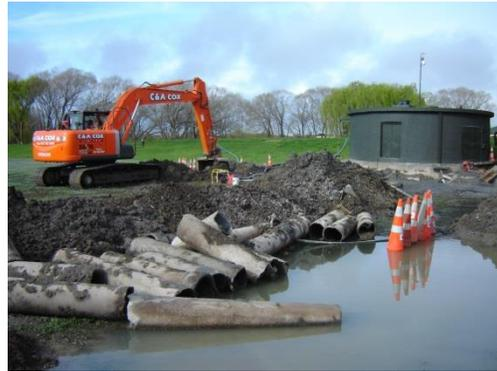
Figure VI – Compression fractures of pipe ends and joints in AC sewer rising main, Charles St, Kaiapoi, axially aligned with the Darfield epicentre, 2010 (Replaced with Biaxially Orientated PVC (PVC-O)
