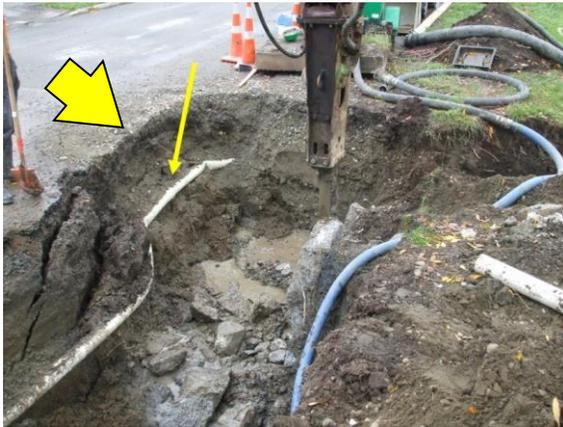
*Figure XI - Distorted but still operational, DN100 PVC-M water pipe with joint, Christchurch*
