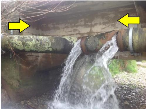
Figure V - Compression distortion and separation of RRJ joints in CLS watermain, 2014
