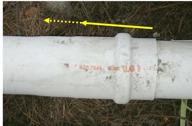
*Figure X – Compressed ductile joint movement in PVC-u water main, Christchurch*
